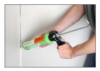
Green Glue Noiseproofing Sealant is a water based acoustic caulk used to seal edges and seams of the drywall and subfloor. Green Glue Sealant can be easily mudded and painted over.
