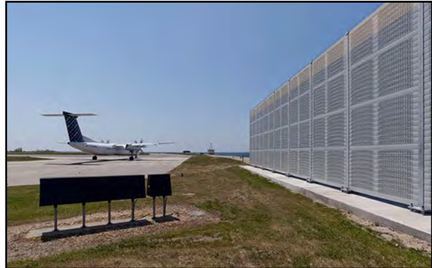
Managing airport noise is a key part of the Toronto Port Authority's commitment to the environment and naturally All Sound Walls were a good fit on this project.
